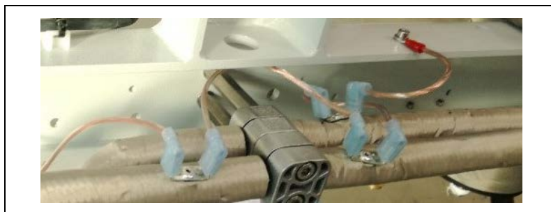
Figure 2.2: Example coating of insulation
