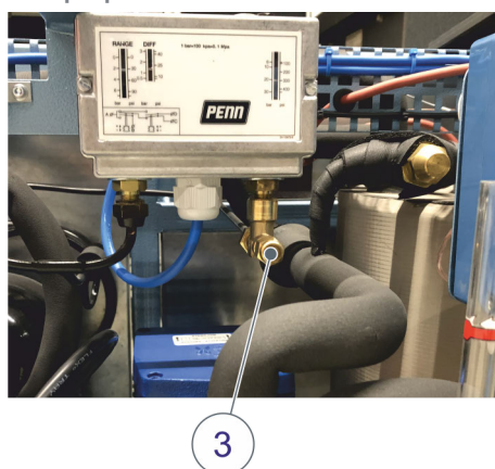
Figure 10.2 Pressure connection on the high-pressure side
